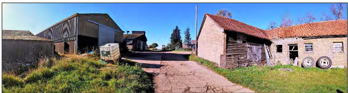
Figure 42: View looking west from Olives Farm in the direction of the PA, with the listed stables/granary block to the right and modern farm buildings to the left
